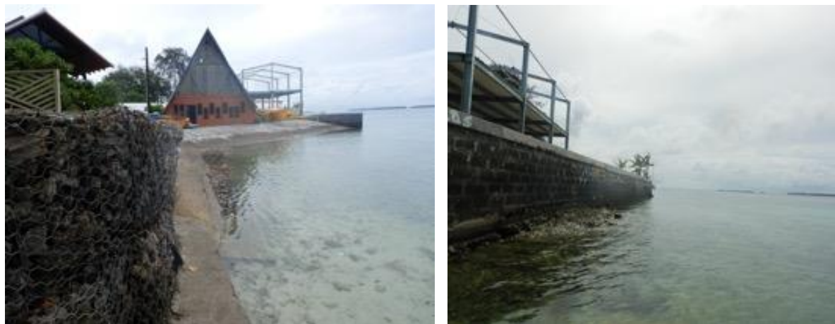
Plate 6: WAM existing seawall
