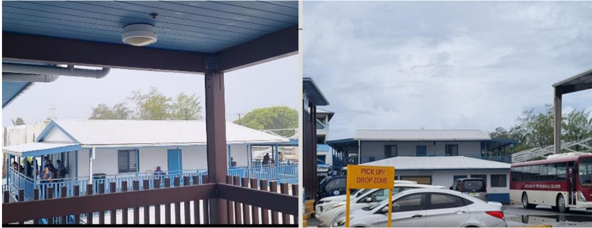
Plate 3: Existing buildings to be demolished at the CMI site
