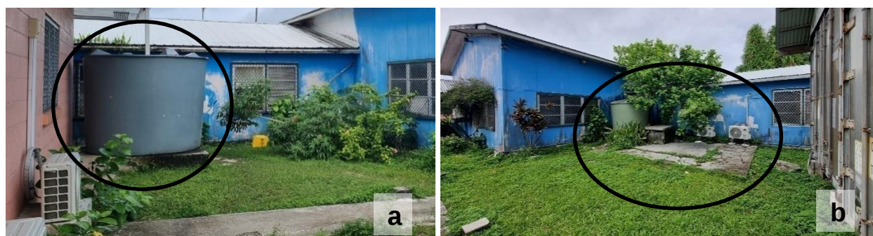
Plate 2: Existing (a) water tank beside the Women's Center ('pink' building), and (b) water tank and septic tank beside the MOEST/PREL Building
