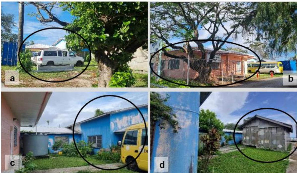
Plate 1: Site photos of Women's Center (a) parked dilapidated cars, (b) MOCIA Women center (pink building), (c) MOEST/PREL building (green), and (d) container (violet).
