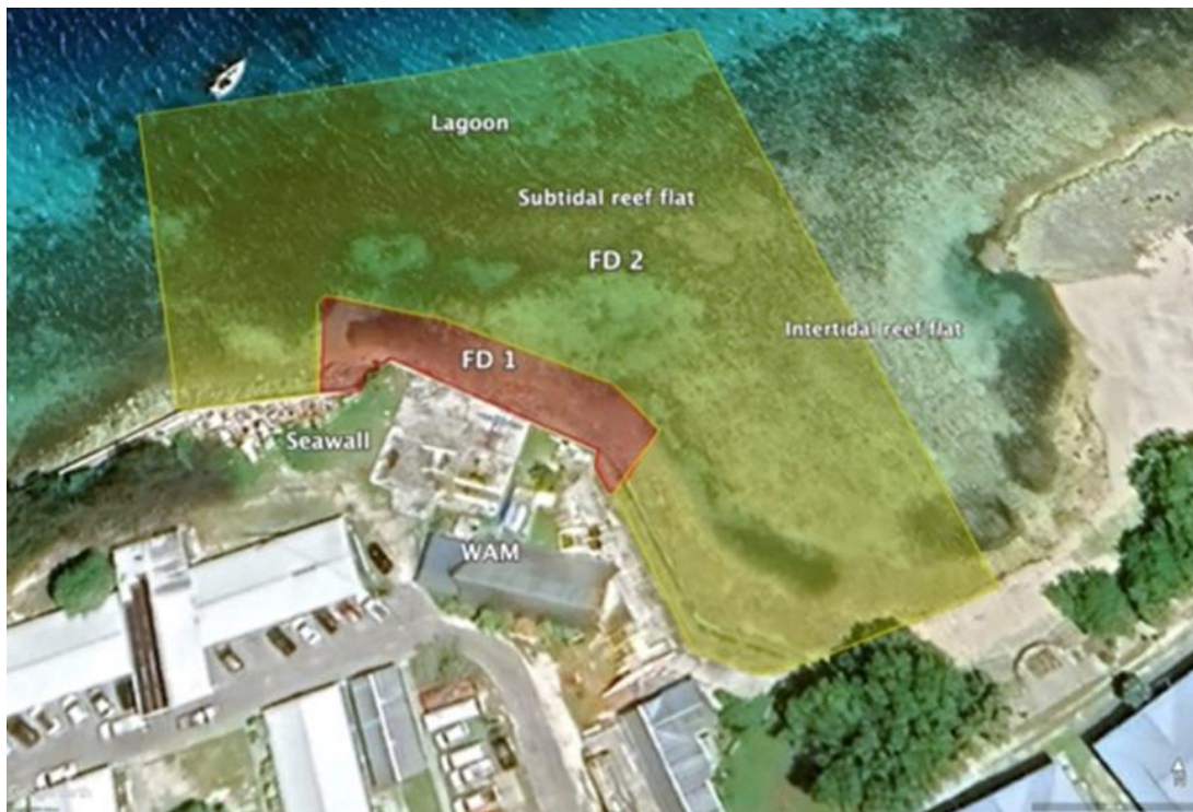
Figure 11: Free Diving sites (FD1 and FD2) assessed for the proposed seawall rebuilding at the WAM site during the marine benthic assessment
