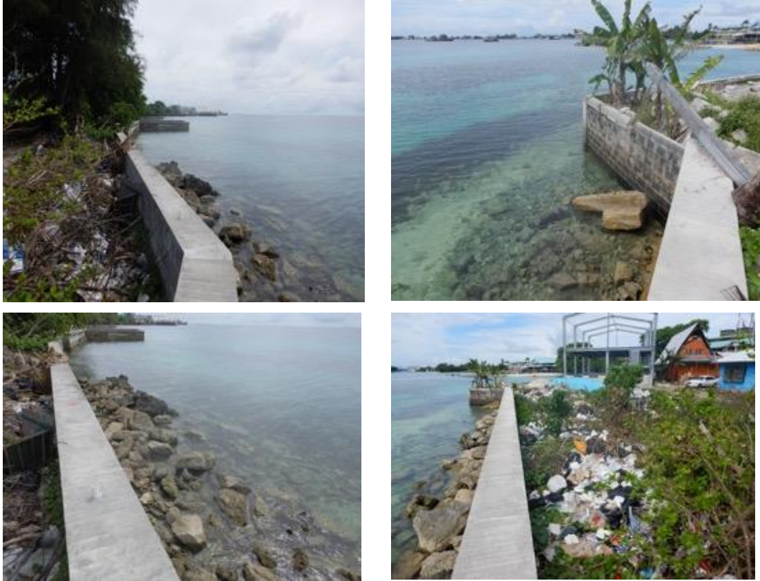
Plate 4: WAM site and associated infrastructure west of the project site.
